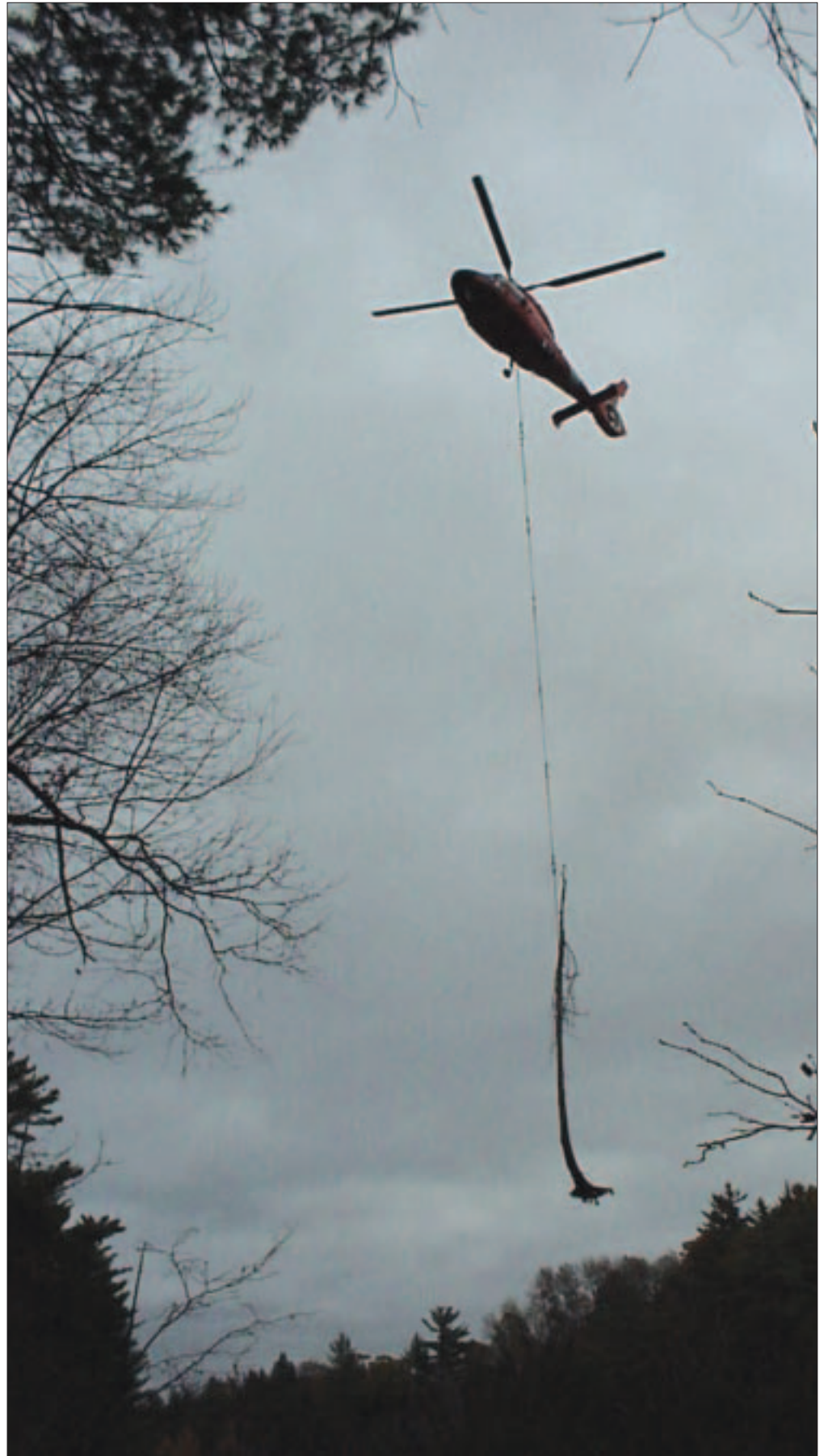
An Air Station Traverse City helicopter hauls a tree to assist in a river restoration project.
